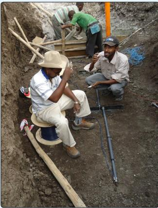
• Fill extensometer array installation
