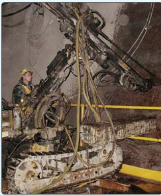
• Borehole drilling for extensometer and piezometer installation.
