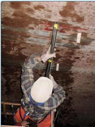
• Extensometer installation.
