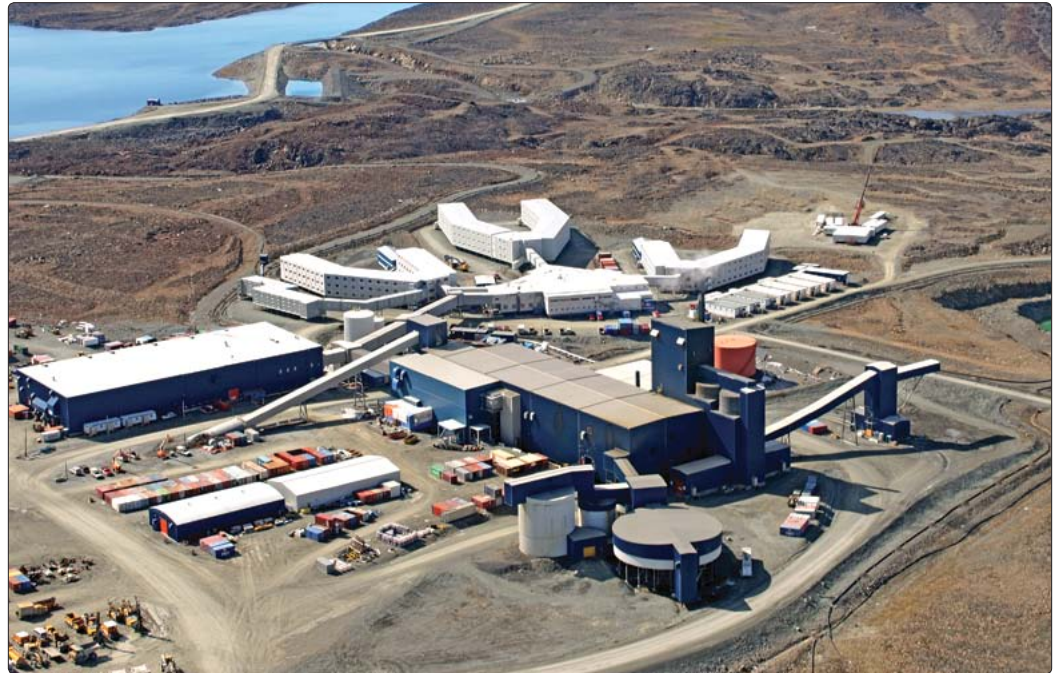
• Raglan Mill plant as seen from above.
