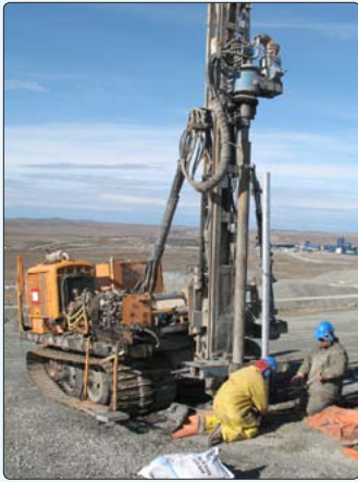
• Thermistor strings, grounding rod and mounting post installation.
