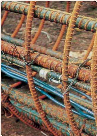
• Close-up of Model 3911 shown as installed in concrete pile reinforcing cage.
