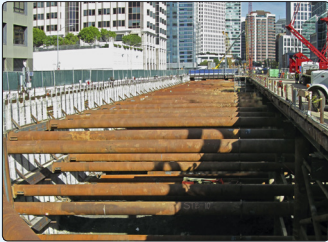
• San Francisco Transbay Transit Center internal bracing system - Excavation zones 1 & 2
