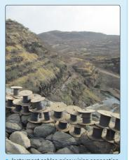
Instrument cables prior wiring connection to data acquisition systems at observation room downstream
