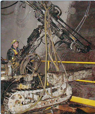
• Borehole drilling for extensometer and piezometer installation
