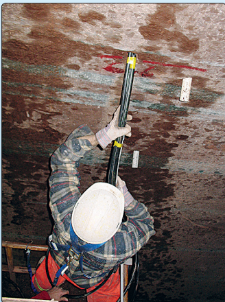
• Extensometer installation
