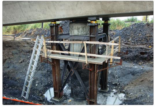
• Lifting support at Pile #2 for bearing device repair
