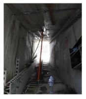
Inclinometer casing being slid through the gallery
