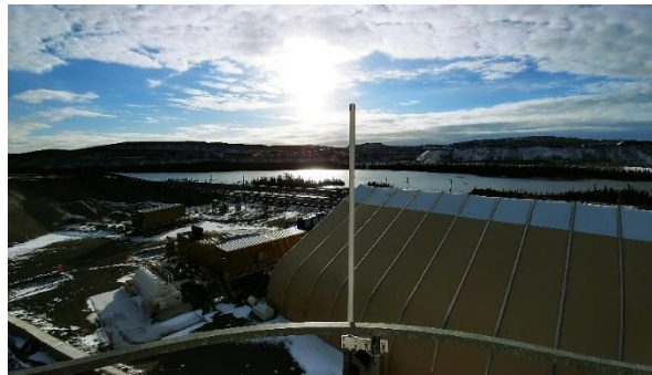
Figure 6 Gateway Antenna installation
