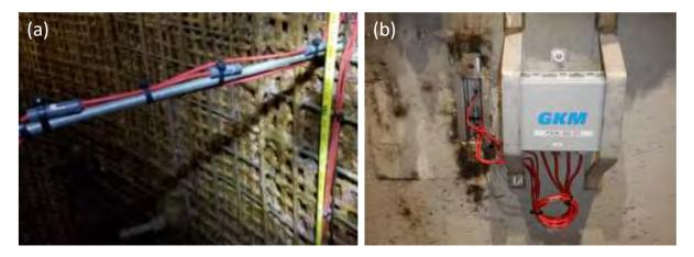
Figure 2 (a) Thermistors attached to their support before the concrete pour. (b) Embedment plate for the thermistors and data logger.
