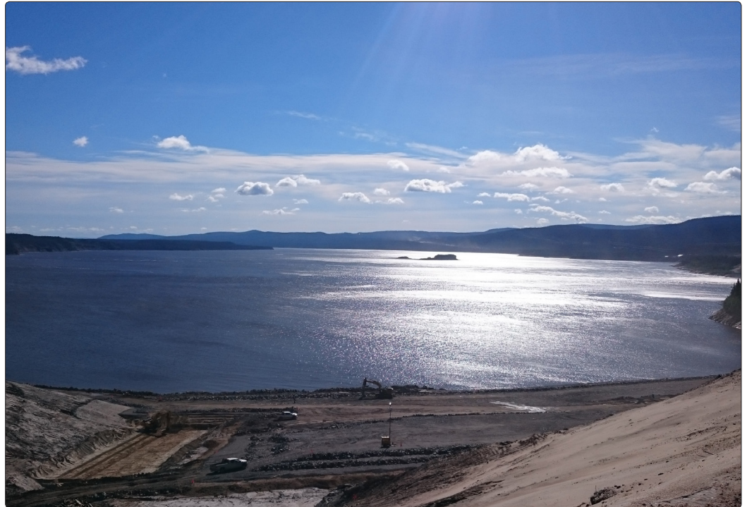
• Muskrat Falls – North Spur, downstream view
