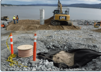
• Standpipe piezometer protection construction
