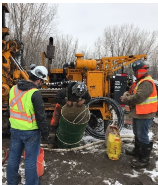
Preparation of grout
