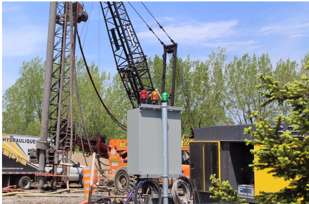
Normandie pedestrian bridge, Longueuil Québec | Vibration monitoring during pile driving
