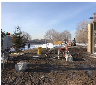
General view of construction site
