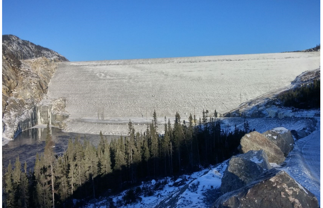
La Romaine-3 Dam, located North of Havre-Saint-Pierre municipality.
