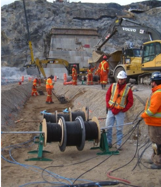
Installation 4500HD piezometers.
