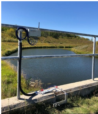
Crack monitoring on the spillway wall
