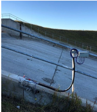
Crack monitoring on the spillway chute
