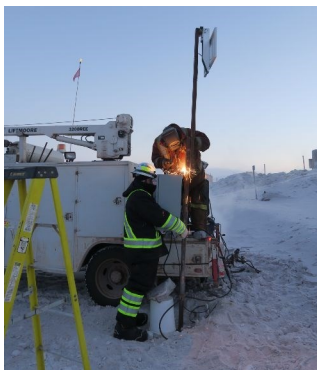
Installation of the casing and solar panel
