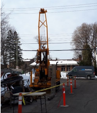
Drilling and installation of multi-point extensometers
