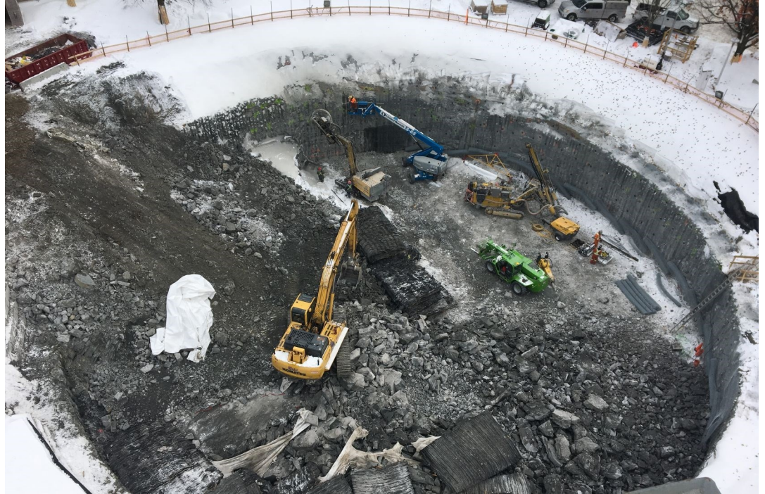
Aerial view of Lavigne flood retention basin excavation
