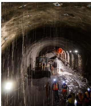
Côte-Vertu garage tunnel – excavation
