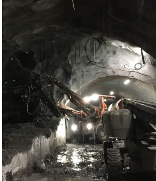
Installation of extensometers in the tunnel
