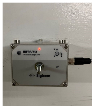
INFRA V12 monitoring vibration
