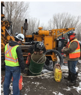
Preparation of grout
