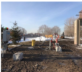
General view of construction site
