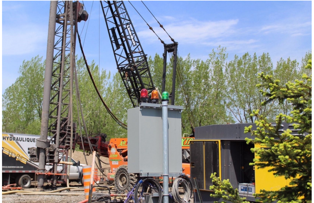
Normandie pedestrian bridge, Longueuil Québec | Vibration monitoring during pile driving
