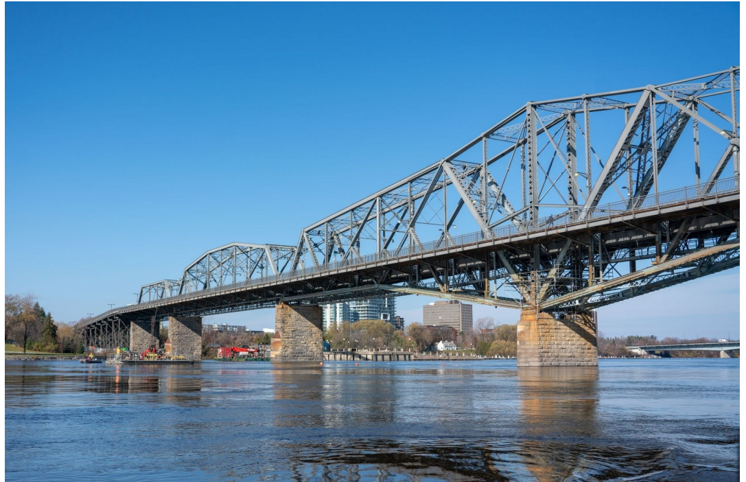
Panoramic view of the Alexandra bridge taken during the installation of our data acquisition systems.
