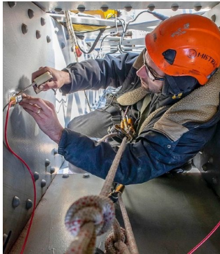
Strain gauges installation on the bridge truss.
