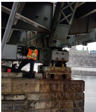
Installation of data acquisition systems under the Alexandra bridge.
