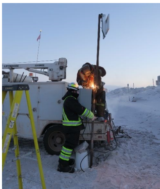
Installation of the casing and solar panel
