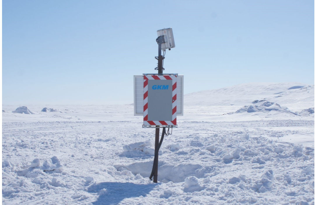
DL series acquisition system with telemetry by satellite antenna
