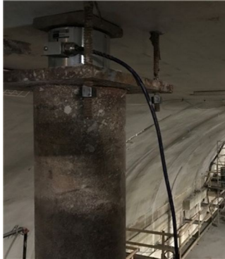
Installing load cells between support struts and the tunnel liner
