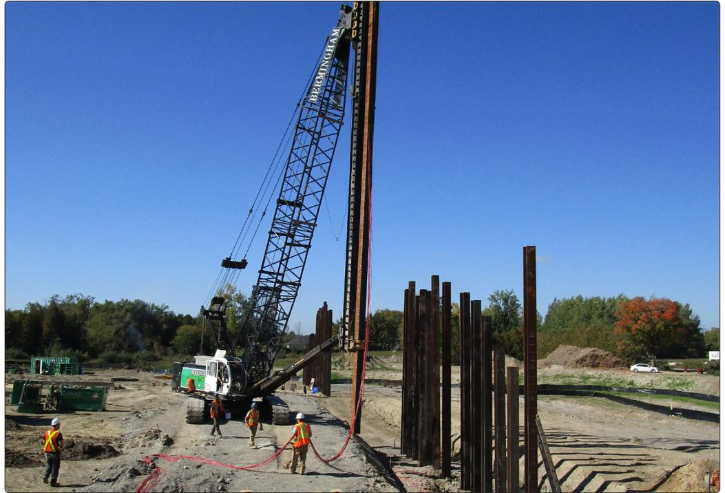
• Instrumented pile being maneuvered into position
