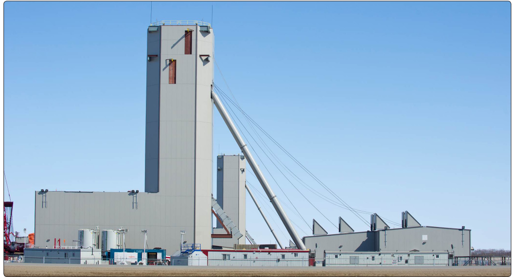
• Production and service shafts view, Jansen Mine, Saskatchewan
