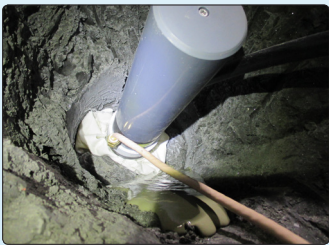
• Ground deformation measurement with Geokon borehole A-3 extensometers
