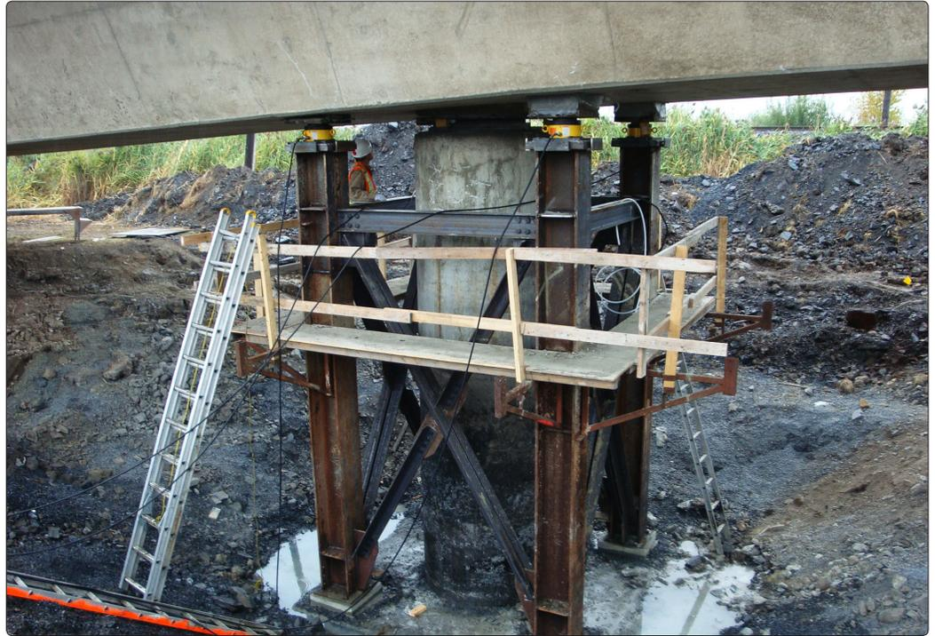
• Lifting support at Pile #2 for bearing device repair
