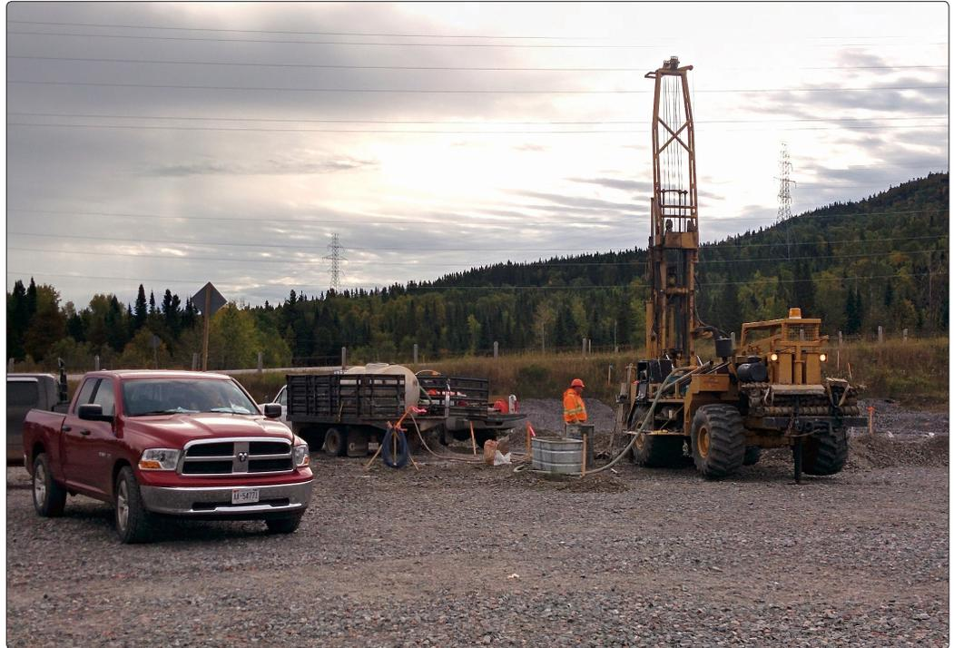
• Piezometer installation in geotechnical boreholes
