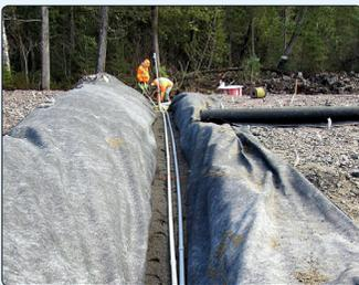
• Shape Accel Array (SAA) installation in horizontal orientation
