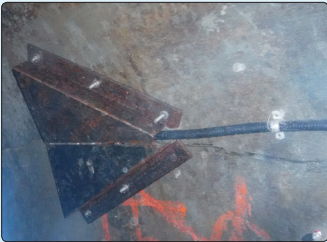
• Heavy-duty protection cover to avoid crackmeters damage from effluent debris
